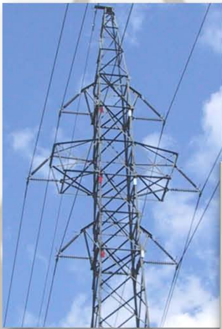
[Applied Iron tower1]
