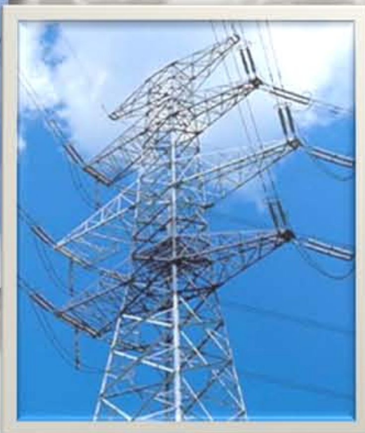
[Applied Iron tower2]
